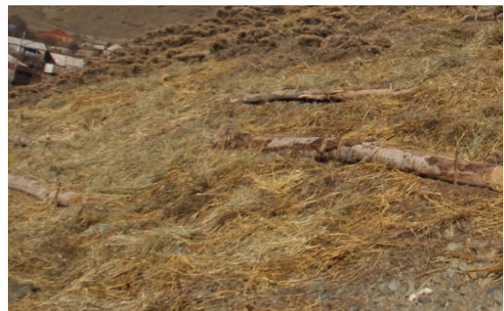
Fig. 5: Pile walls and mulching are applied to combat advanced sheet erosion on a slope.
