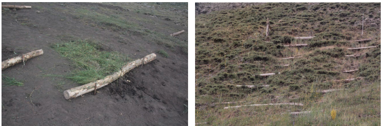
Fig. 5: Examples of pile walls on different pilot sites. Offset establishment of pile walls (left) and below each other in water run-off grooves.
