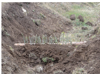
Fig. 5: Forming terraces by filling the space behind the wooden log and the willow cuttings with soil.
