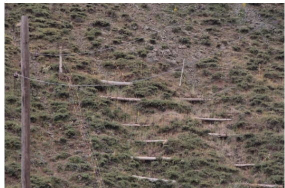
Fig. 6: Pile walls to combat rill erosion
