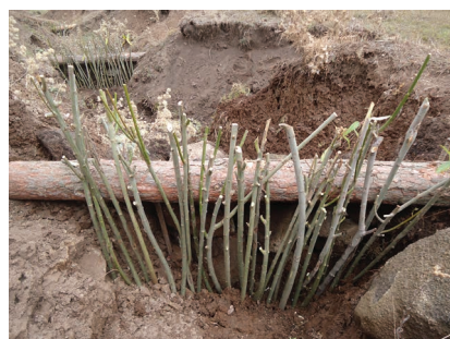
Fig. 4: Placing of tree cuttings behind the wooden log.
