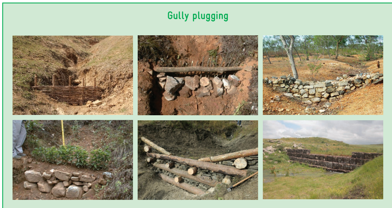
Fig. 7: Gully plugs constructed with different materials
