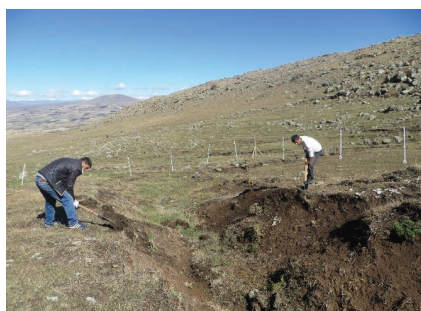
Fig. 3: Flattening of gully shoulders.
