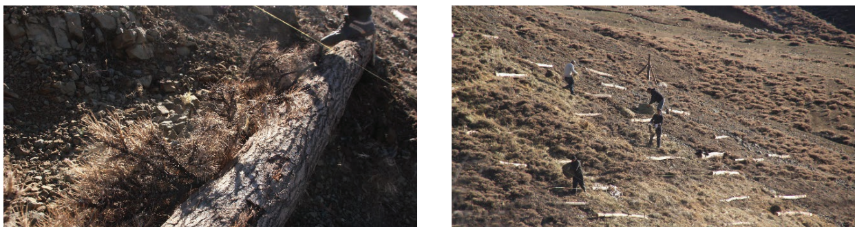
Fig. 4: Filling up the area behind the wooden log with soil and plant material (left) and covering open soil with hay (right). November 2016.
