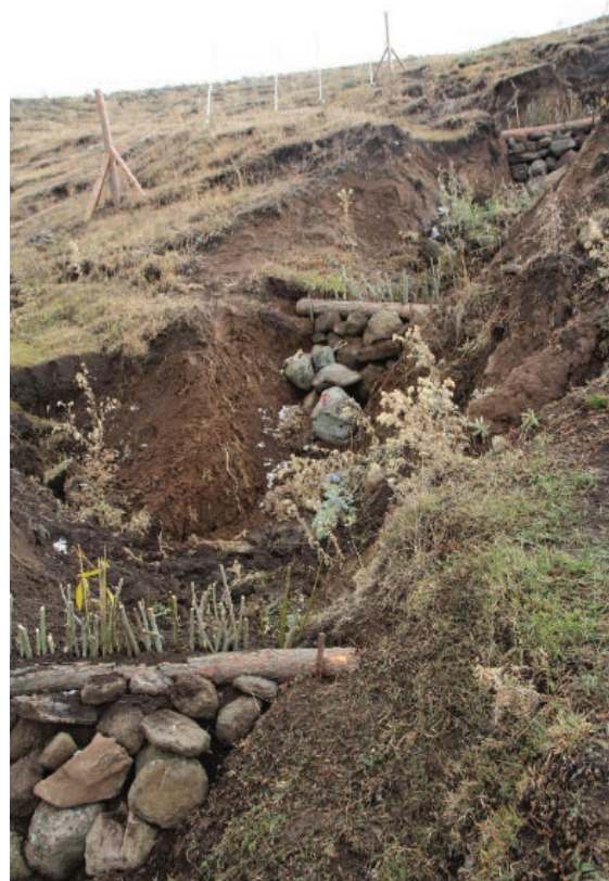
Fig. 7: Check dams to slow-down water movement in gully.
